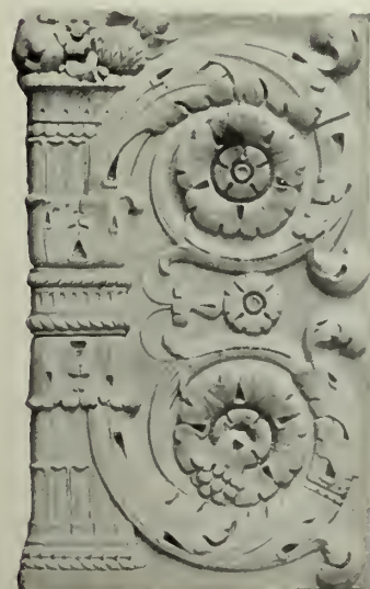
DETAIL BY CROW, LEWIS & WICKENHOEFER, ARCHITECTS. Executed by the Conkling-Armstrong Terra Cotta Company.
